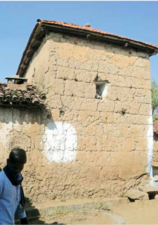
This page, top: a typical Medak house with cob walls over 3' granite stone walls. Left: intricately carved Neem wood brackets. Below left: play of the roof scapes of hollow interlocking clay tiles. Below right: a G+1 cob house showing horizontal bands
