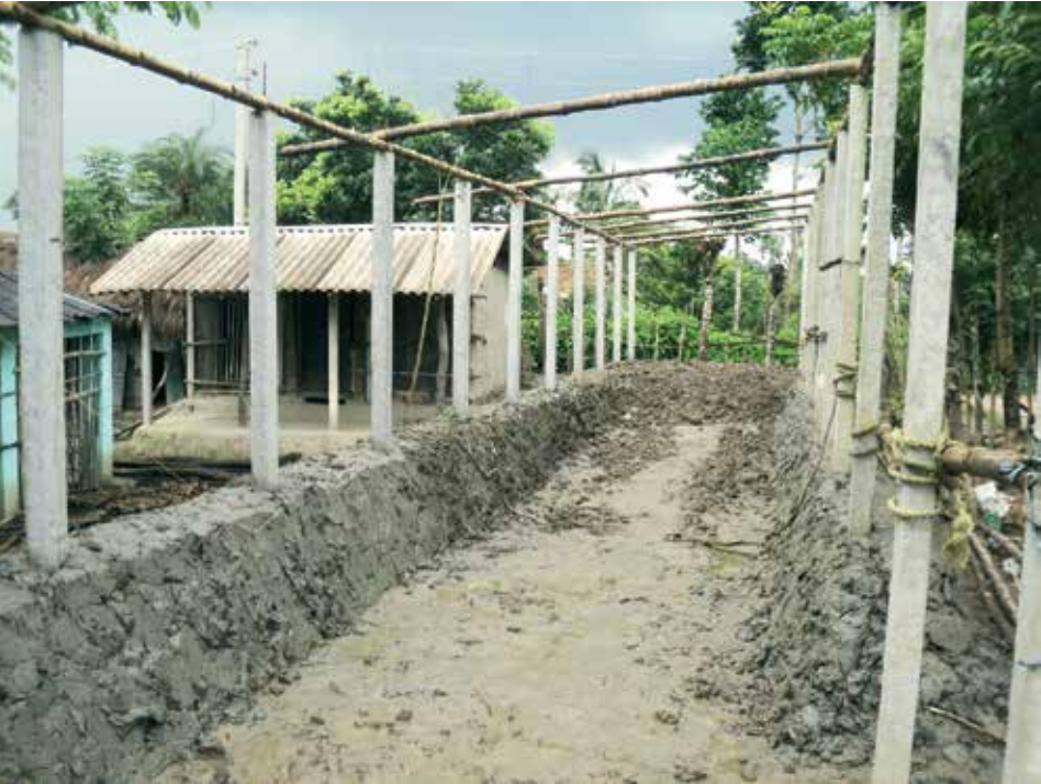
This page, left: pre-cast RCC posts for the house frame anchored in mud. Below left: rice paddy straw thatch. Below right: periodic flooding causing erosion and damage to mud plinth. Far below right: a typical Wattle and Daub house
