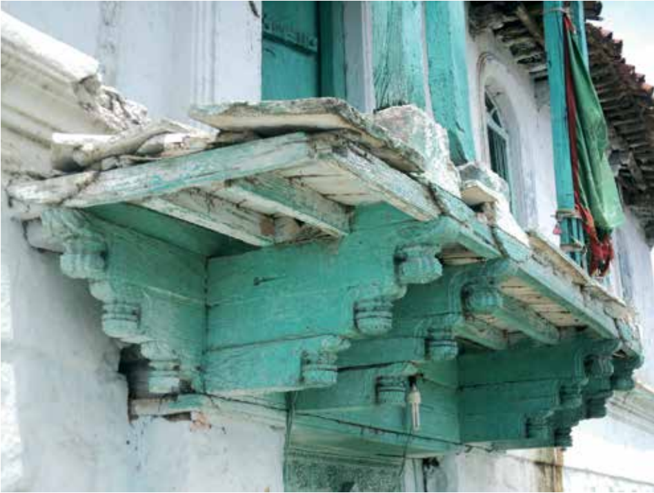
This page, top: a typical Medak house with cob walls over 3' granite stone walls. Left: intricately carved Neem wood brackets. Below left: play of the roof scapes of hollow interlocking clay tiles. Below right: a G+1 cob house showing horizontal bands
