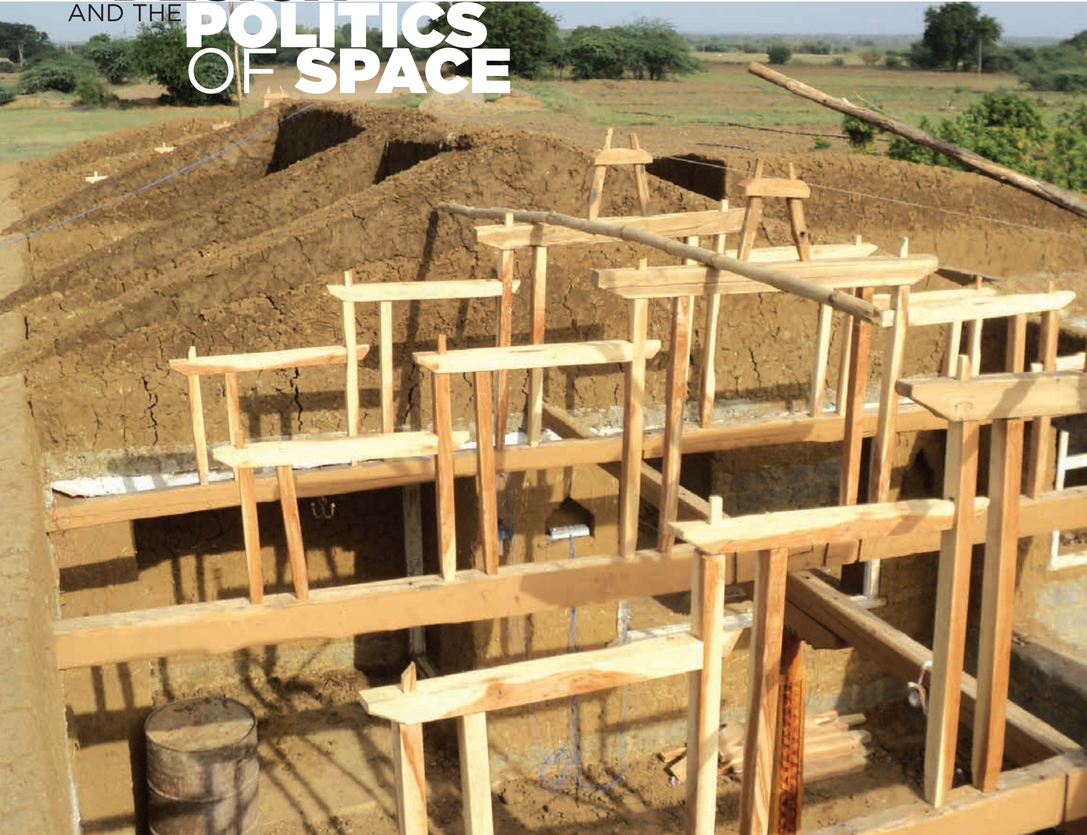
← Intricate Neem wood roof trusses, Yakshi Learning Centre, Medak District, Telangana
