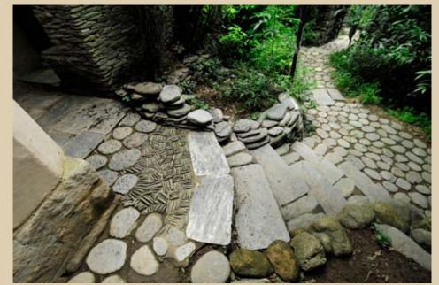
Left: Slate, a common building material in the area is used for floors, steps and roofing. Pathways are paved with slates shaped by the near by river. Large river gravel, organized in a pattern at the entrance, forms a natural doormat.
