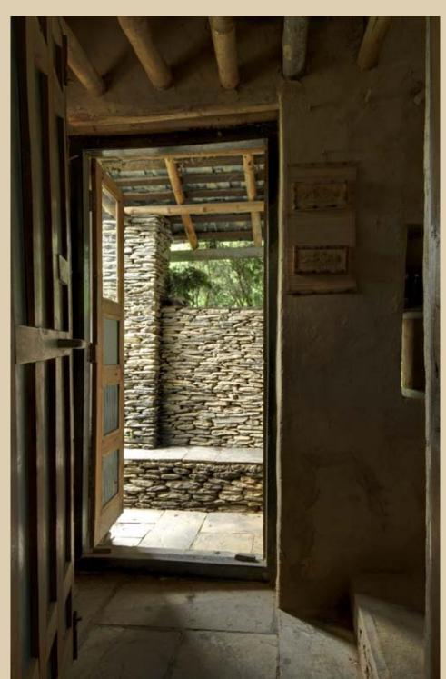
Left: The entrance porch is created with stacked stone with a part of the wall broadened at the base to form a seat. Slate moves up one level and becomes the surface of the seat. Stacked stone masonry is one of the elements of the Himachal vernacular. Didi re-interprets it in her buildings in a designed manner.
