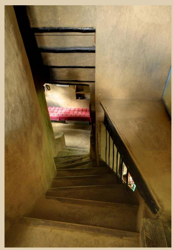
Left: Transition from one level to another is treated with the same attention to detail and Didi spends a lot of time designing her staircases. Visual connections are retained and the steps are reinforced with treated timber.
