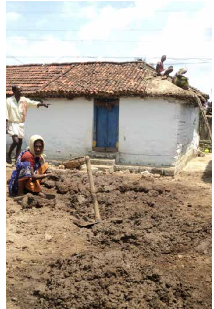
Cob mud balls being prepared from the loamy mix
