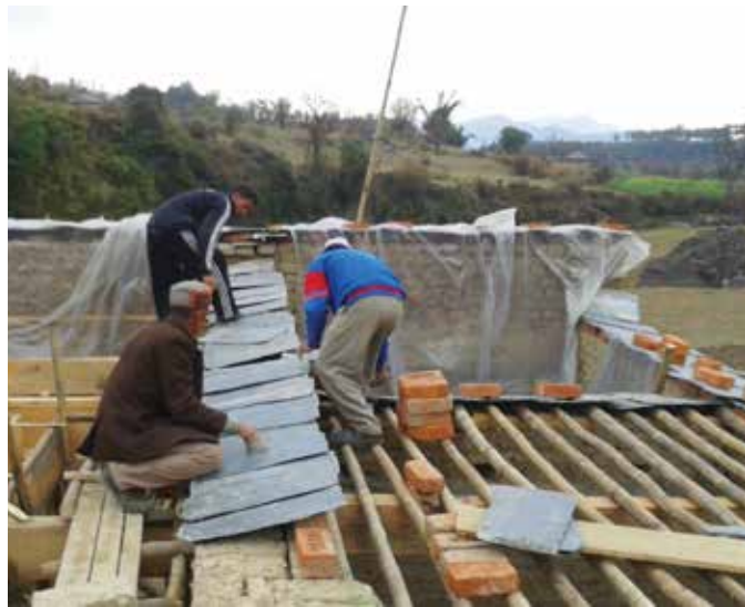
Covering adobe walls to protect from rains
