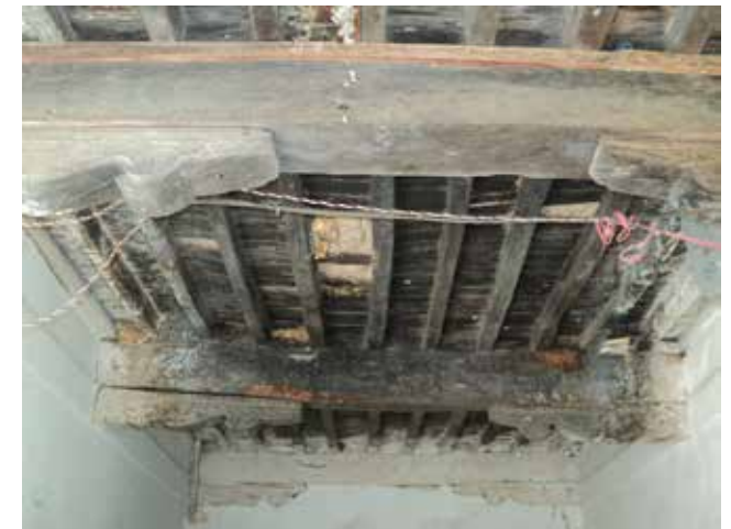
Intermediate roof of Neem wood beam, joists and battens
