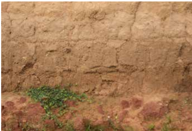
Cob walls over laterite stone foundation
