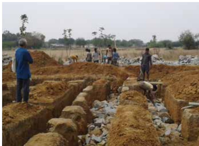
Random rubble for foundation with mud mortar
