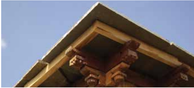
Corner bracket detail in Neem wood
