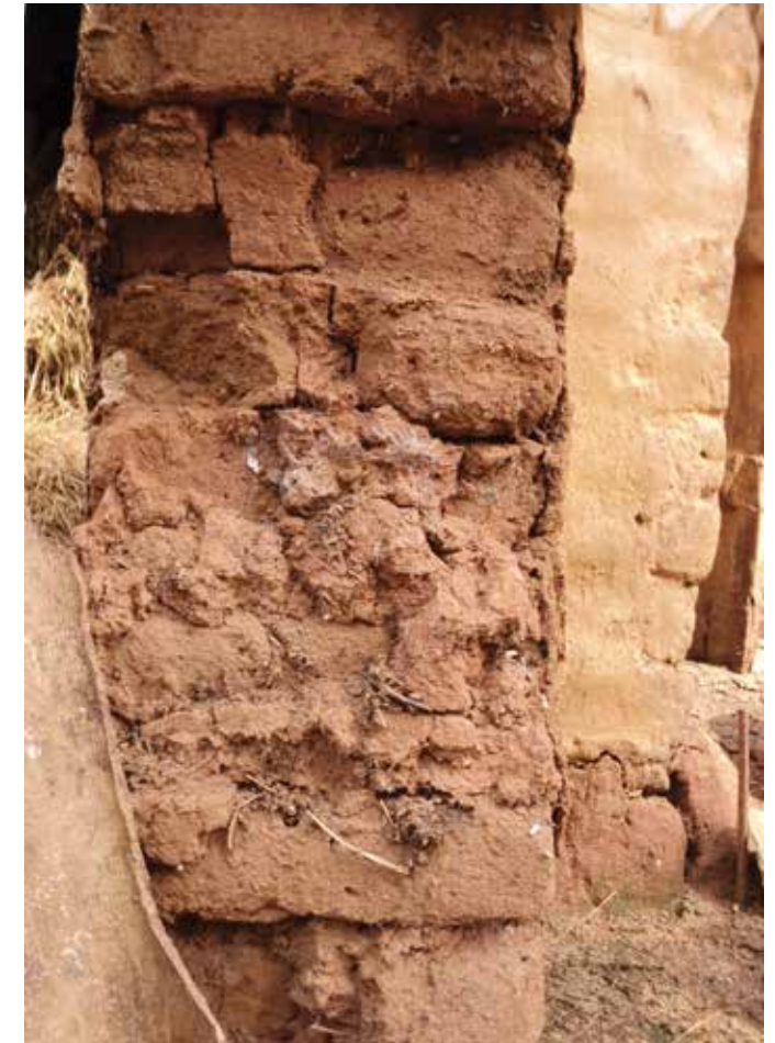
Adobe walls of 1foot thickness with mud mortar
