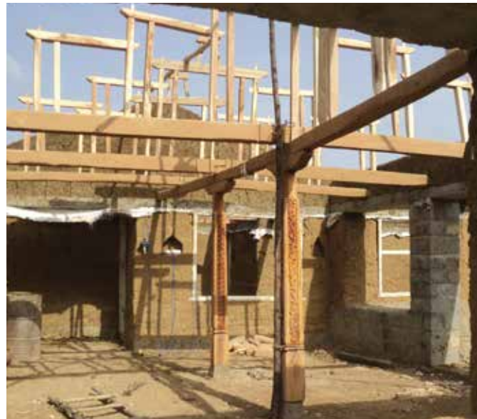
Rooftruss with carved Neem wood pillars
