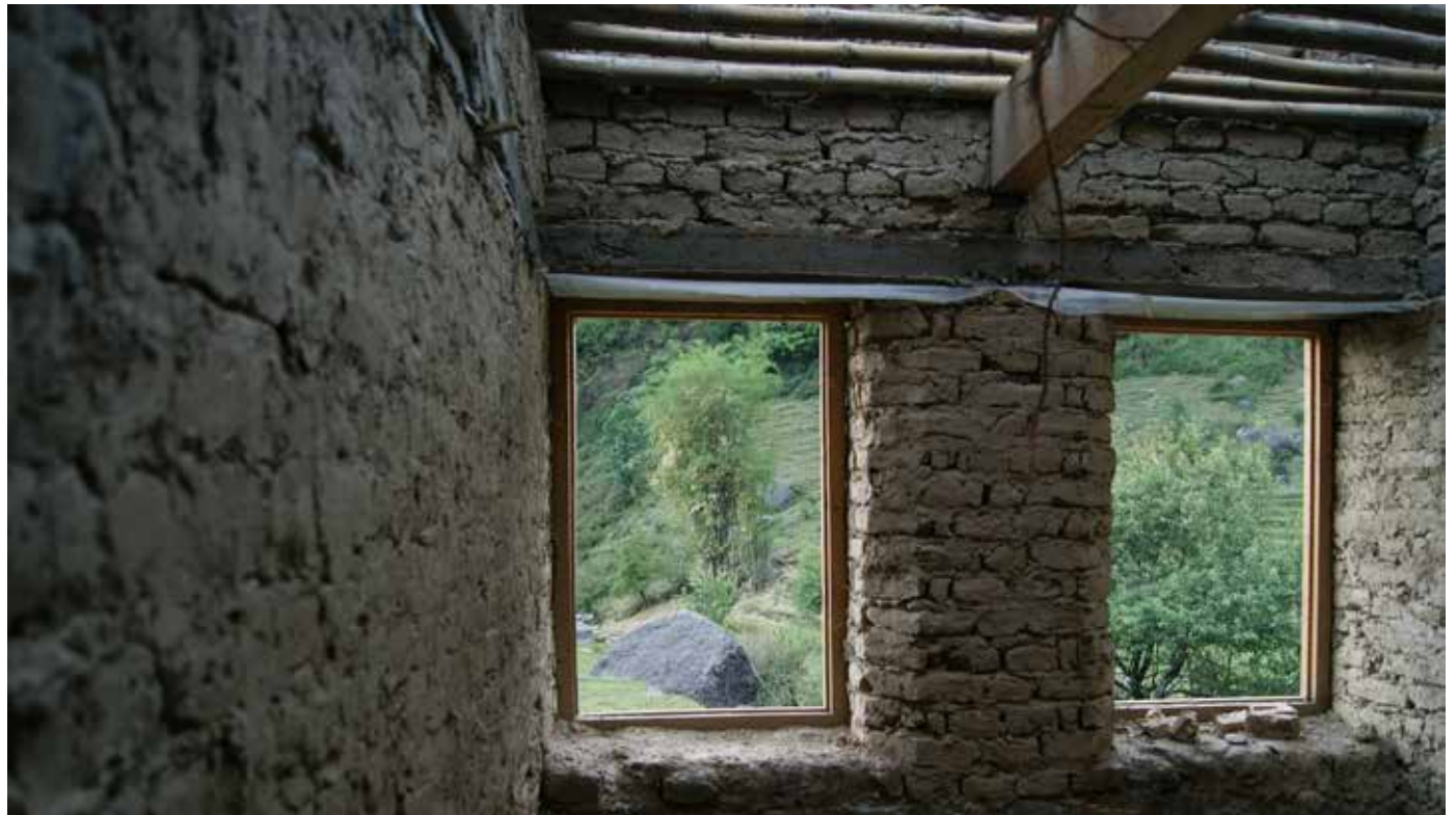
Adobe walls and bamboo rafters over pine wood beam
