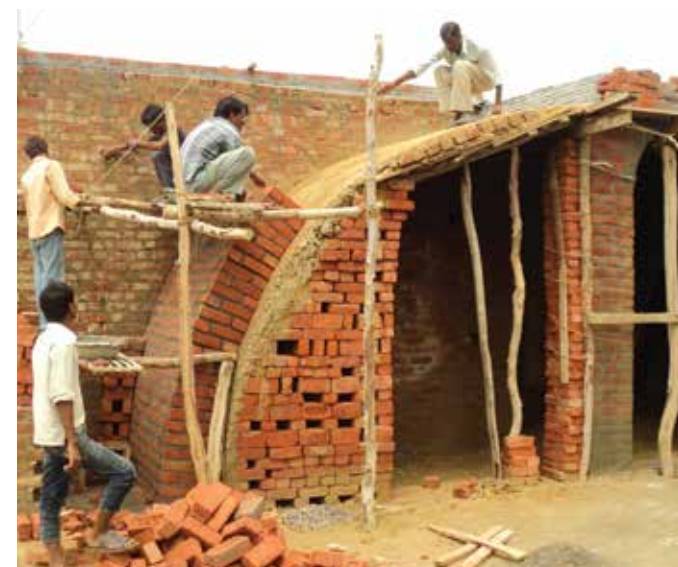
Building a 12 foot span brick masonry vault for stairs above
