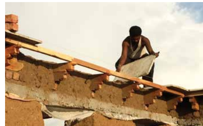
Carpenter Santosh fixing shahbad stone overhangs or chajjas
