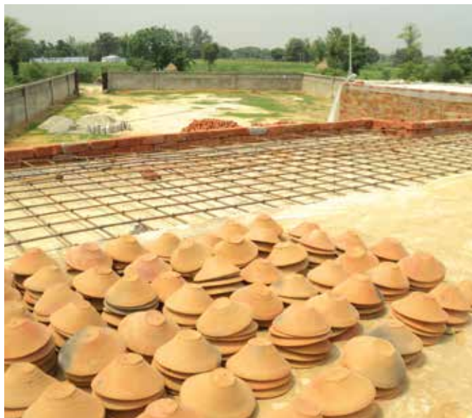
Clay pots used in R.C.C filler slab
