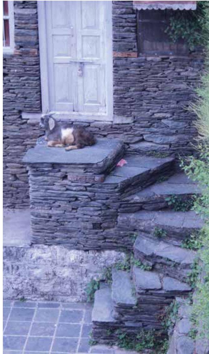
Dry stack masonry walls
