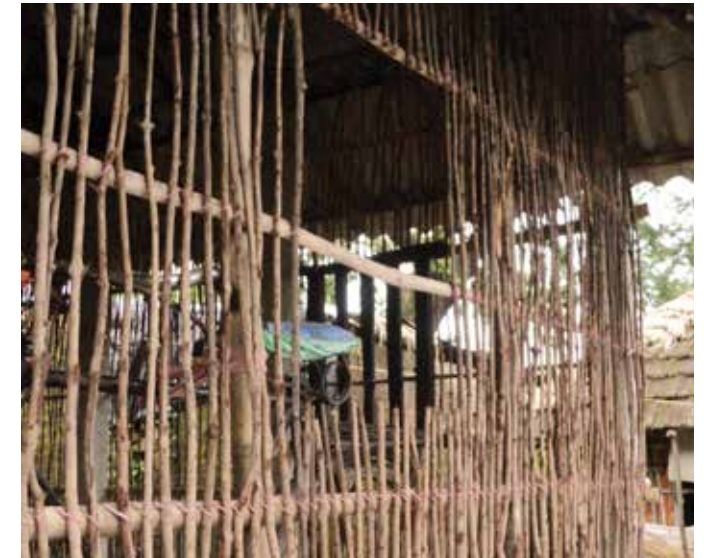
Wattle made of branches of the Sundri tree
