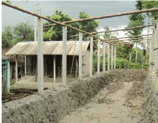
Pre-cast RCC posts for the house frame anchored in mud
