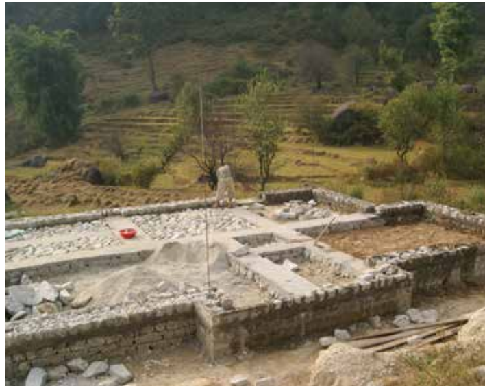
Foundation and plinth in local dressed stone
