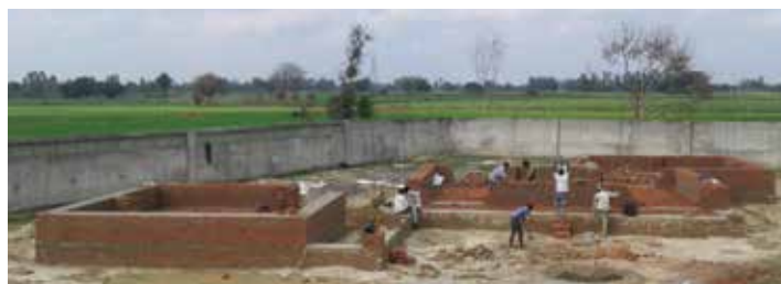
Baked brick external walls upto cill level
