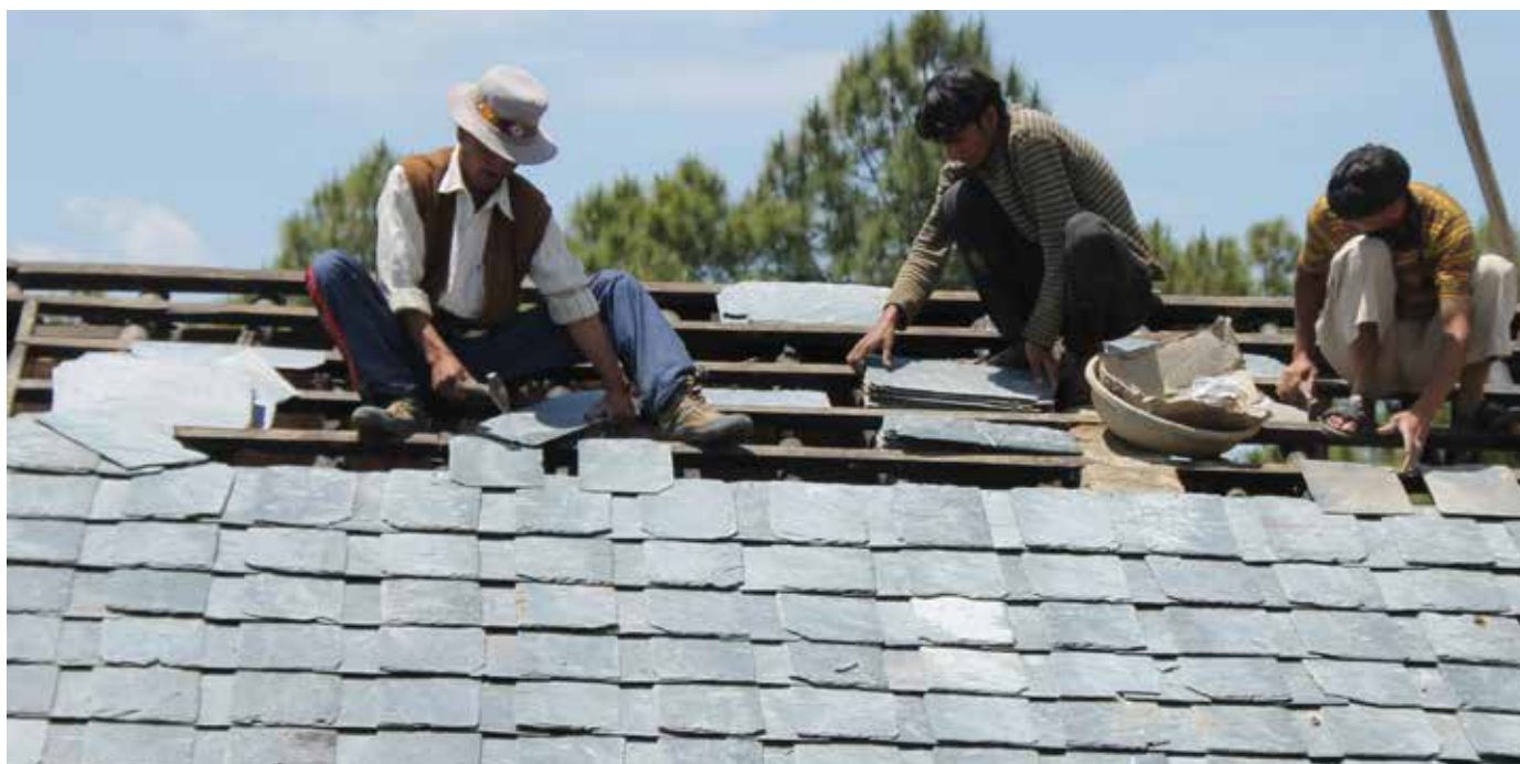
Chamaar and Lohaar carpenters fixing slate over verandah roof
