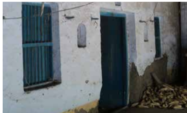
Adobe walls with lime plaster
