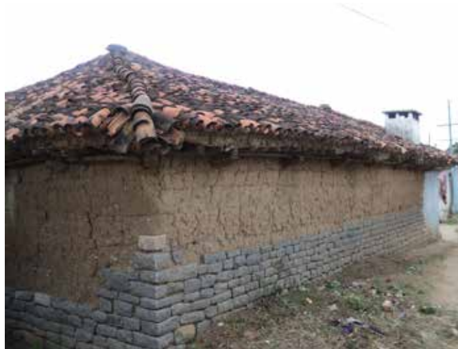
A typical Medak house with cob walls over 3 feet high granite stone walls
