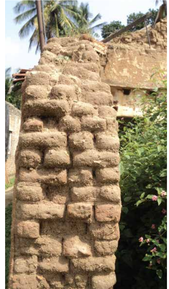
Adobe Walls Section showing 18inch thickness
