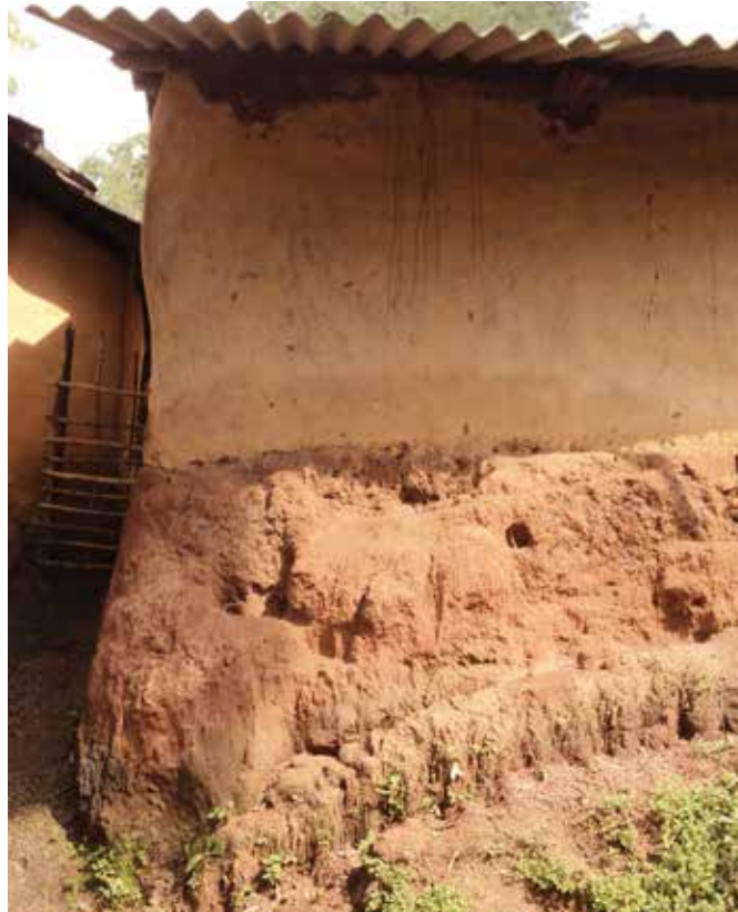
Red laterite stone and mud for foundation and plinths
