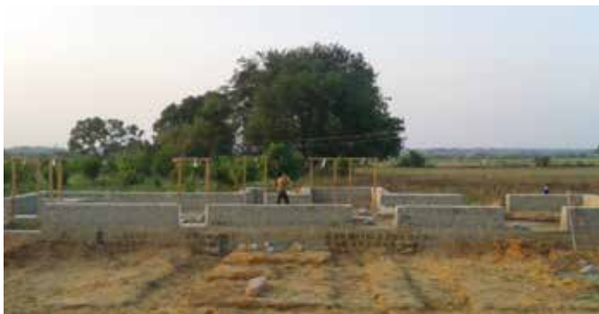
External walls in granite upto cill level
