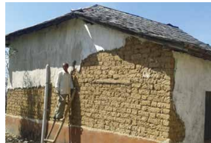
Adobe used for walls above window cill level
