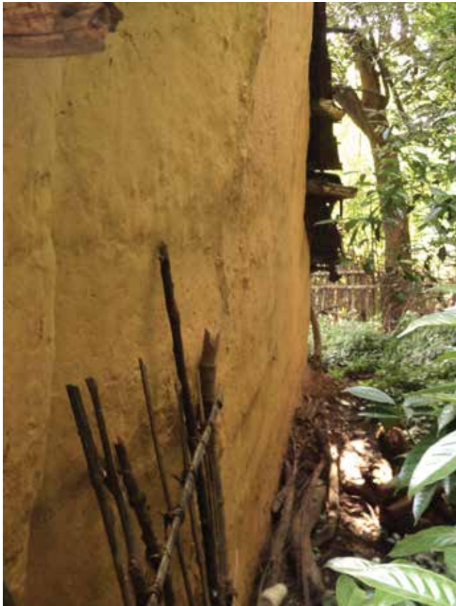
External walls plastered with mud and natural dye pigments
