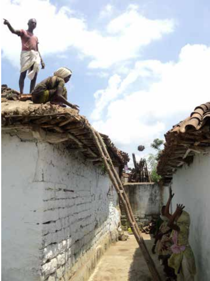
Cob balls being thrown up to the master mason
