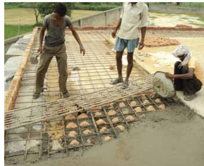
Laying of cement-concrete mix over clay pots
