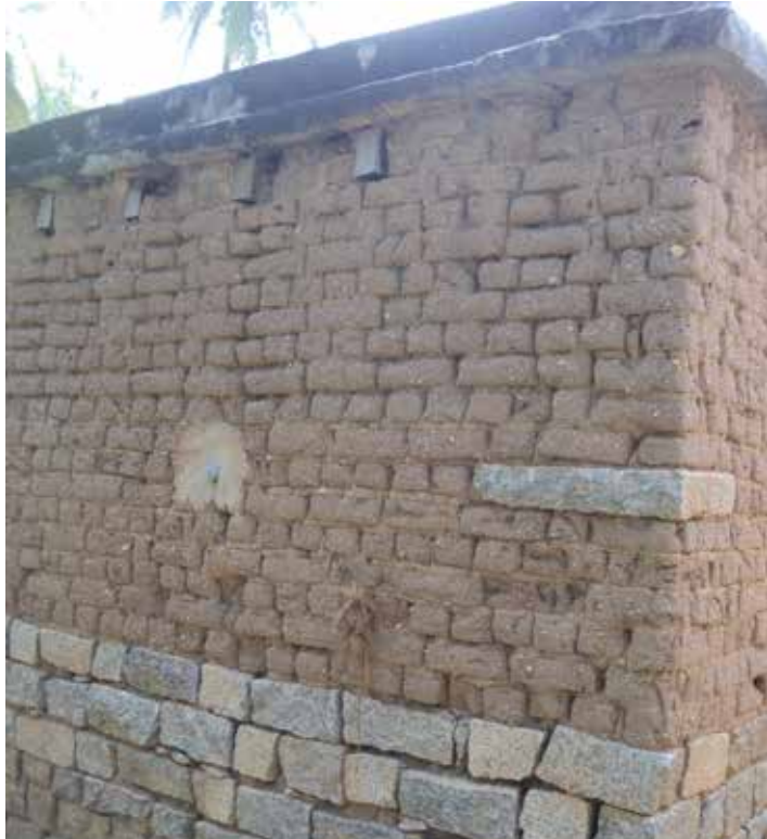
Adobe walls with granite corner stone for adequate distribution of load and breaking of vertical joints
