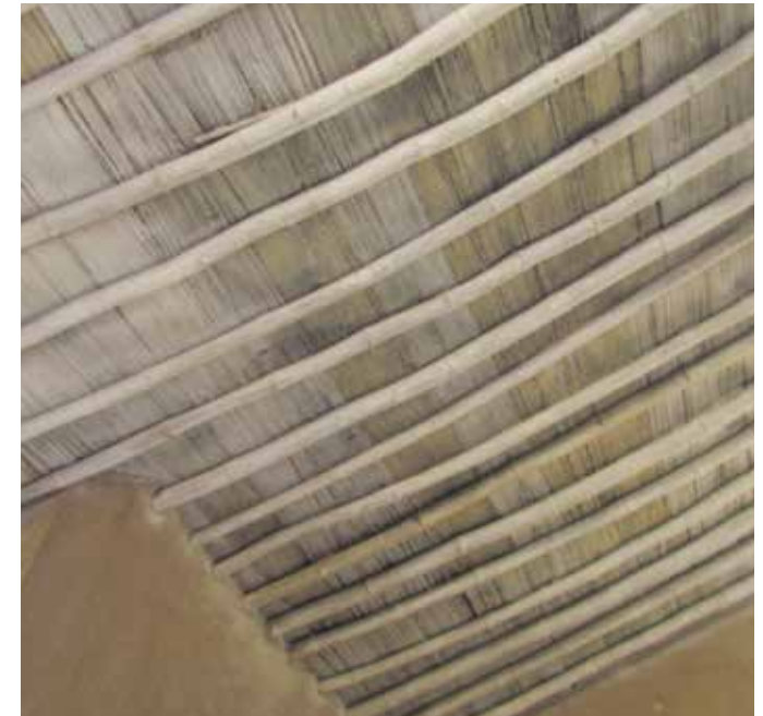
Bamboo and split bamboo roof underbelly
