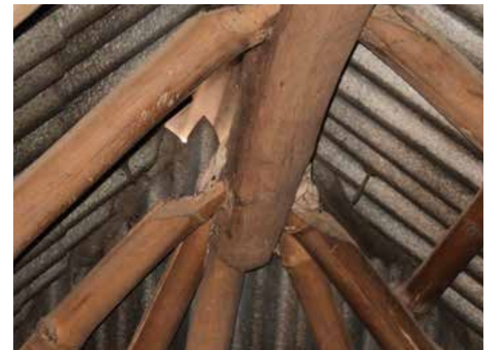
Detail of joinery between mahua wood ridge and bamboo rafters
