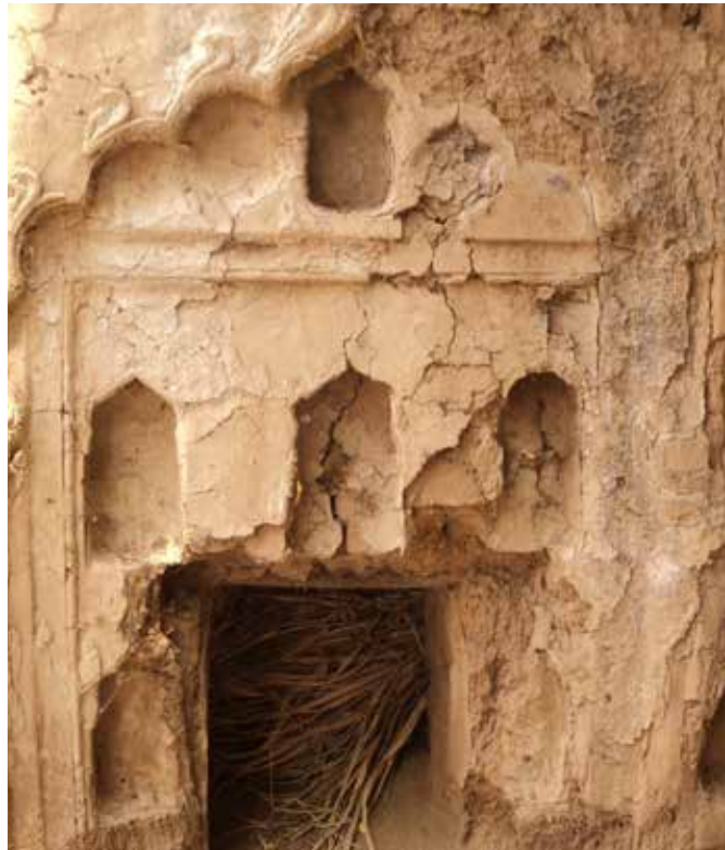
Adobe wall with alcoves and niches to maximize space
