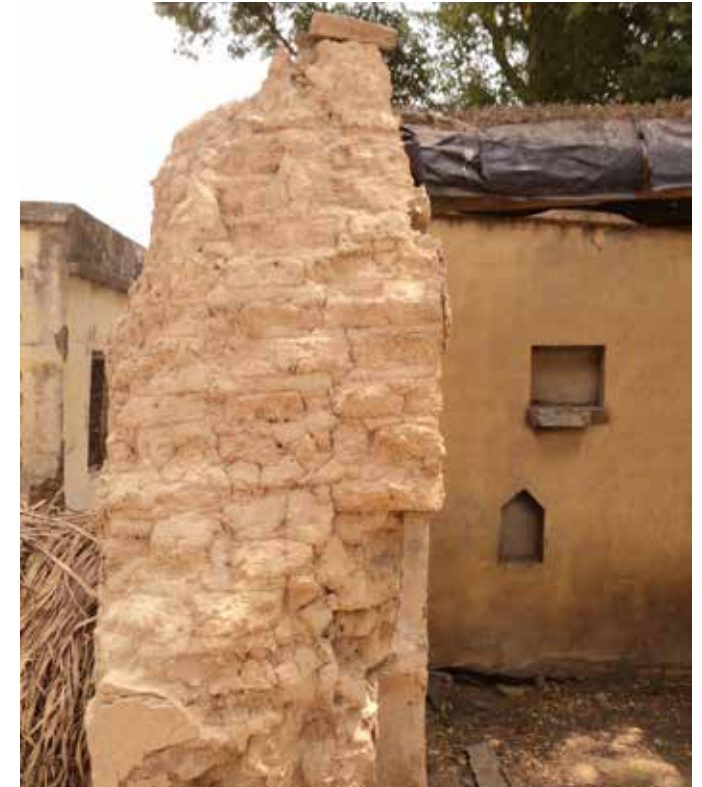
Adobe wall section showing 27 inch wall thickness
