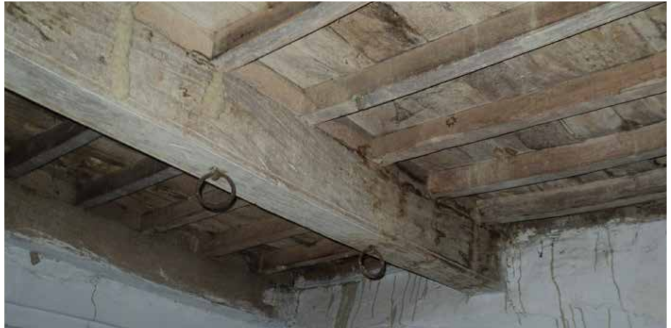
Flat Roof of Neem wood beam, joists and battens
