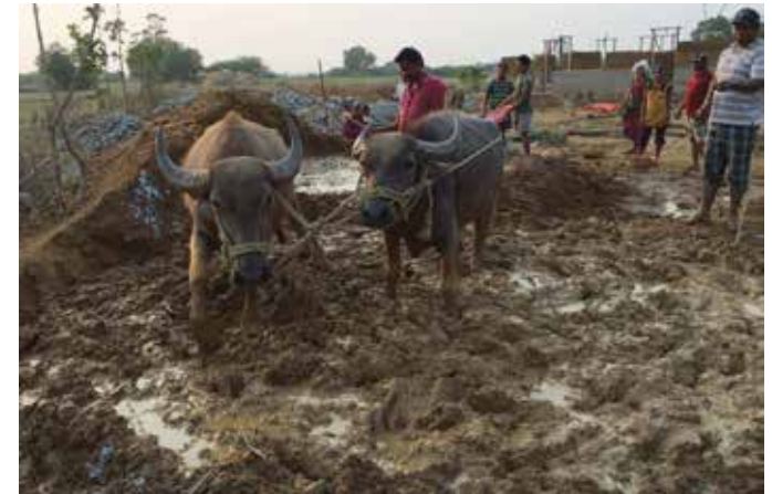
Buffaloes mixing mud, lime slurry and water for cob walls
