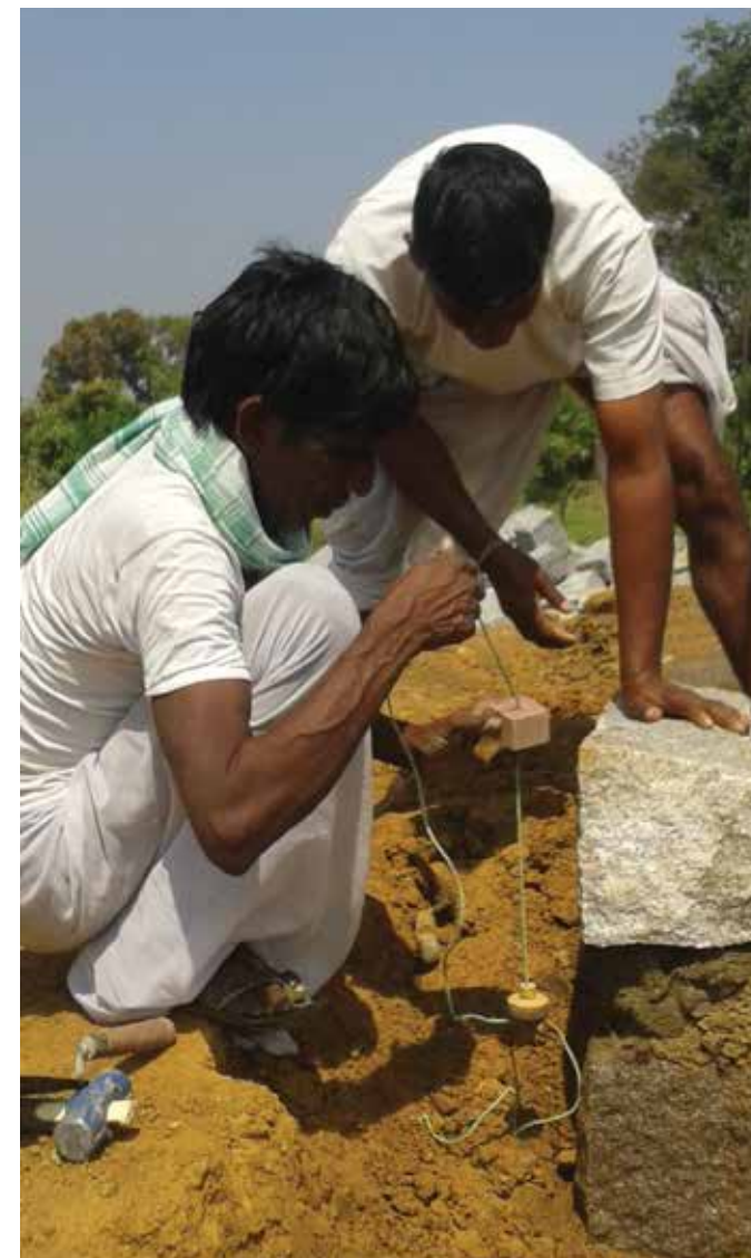
Masons checking plumb line of granite plinth
