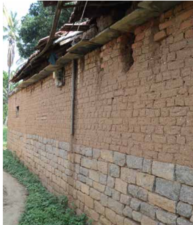
Adobe walls over 3 feet high impervious granite stone walls.
